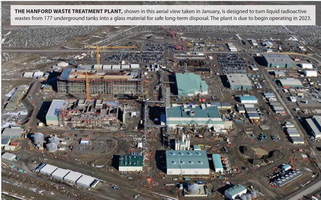
**THE HANFORD WASTE TREATMENT PLANT**, shown in this aerial view taken in January, is designed to turn liquid radioactive wastes from 177 underground tanks into a glass material for safe long-term disposal. The plant is due to begin operating in 2023.
